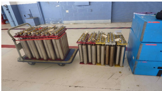
Modules ready for installation.
