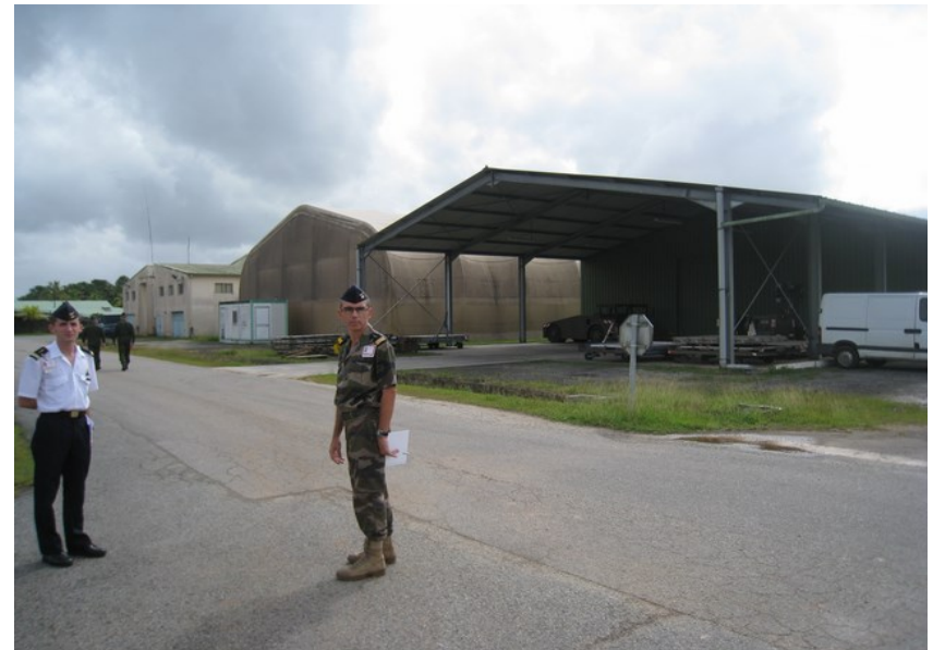
Falcon hangar (white) from the car park
