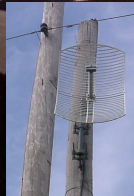
Utility pole (AAMU)
