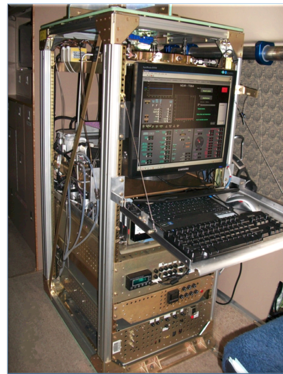
TOGA installed on GV
